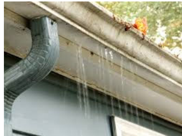
Gutter overflow
