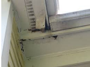
Soffit damage
