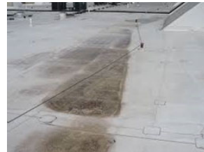
Vegetation growing on roof Stains from pooling water
