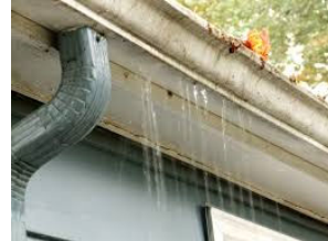
Gutter overflow
