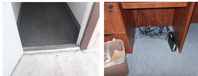
Common office trip hazards
